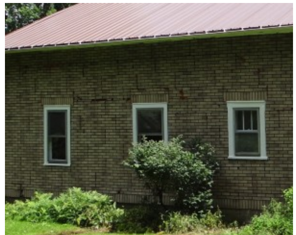
Repainted Windows and Sash on an Old House
